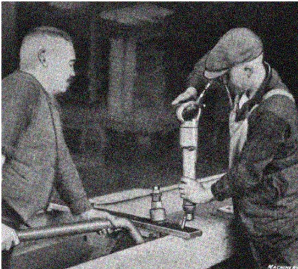
Dolly-bar used as lever for Holding-On
